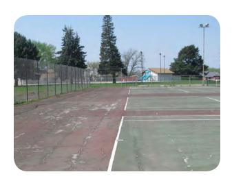
Playing Surface is severely cracked or uneven and needs to be replaced; Drainage issues leave the court susceptible to major pooling of water that regularly limits play; Lighting Fixtures (if present) mostly need repair or replacement; evening play is not possible; Enclosure (if present) is damaged in most sections, some sections may be missing; the loss of tennis balls is common and affects play.
