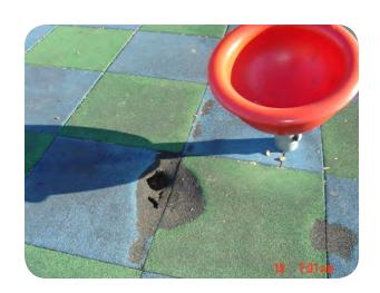
Play Equipment is damaged in parts or missing minor pieces but the majority of the equipment is usable and compliant with safety standards. Safety Surfacing is installed where recommended but may need repair or replenishment to meet safety standards. Edging and borders only partially contain loose materials. Drainage issues create muddy areas or pooled water appear after a rain, but use is rarely affected.
