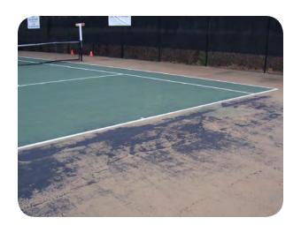
Playing Surface is playable but has some cracks, a slightly uneven surface, or paint that is chipped and worn. Net supports may be leaning but still hold up the net; Drainage issues leave the court susceptible to pooling of water that occasionally limits play; Lighting Fixtures (if present): need some repair or replacement; evening play is possible but uneven lighting affects play; Enclosure (if present) is damaged in some sections, resulting in the occasional loss of tennis balls.
