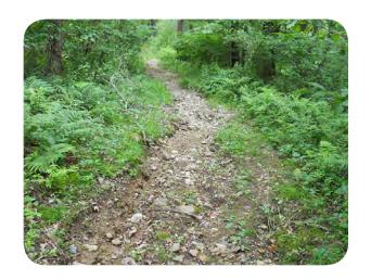
**Surface** is uneven, with signs of wear and minor erosion on unpaved trails and cracks or damage on paved trails. **Signage** has damage or graffiti that affects its legibility. Poles are leaning or are unstable. **Drainage** issues cause some trail erosion during rain; muddy areas or pooled water appear after a rain, but use is only occasionally affected.
