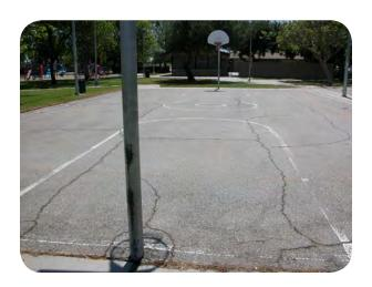
Playing Surface is playable but has some cracks, a slightly uneven surface, or markings that are chipped, worn, or missing; Hoop Supports lean or are slightly unstable and/ or the backboard is damaged to the point that play is affected; Drainage issues leave the court susceptible to pooling water that occasionally limits play; Lighting Fixtures (if present) need some repair or replacement; evening play is possible but uneven lighting affects play.
