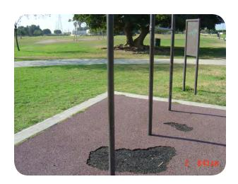
Equipment is mostly in good repair and fully usable; footing may be slightly exposed, but generally undamaged, required repairs are minor and do not prevent use; Instructional Signage is damaged, but is still mostly legible, footing may be slightly exposed; Paths/Ground Surfaces are slightly uneven, with depressions around equipment that expose footings, allow small amounts of water to pool and may limit access for some users.
