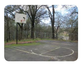
Playing Surface is severely cracked or uneven and needs to be replaced; Hoop Supports are unstable, damaged or missing; post footing may be damaged; post needs replacement. Play is severely limited; Drainage issues leave the court susceptible to major pooling of water that regularly limits play; Lighting Fixtures (if present) mostly need repair or replacement; evening play is not possible.
