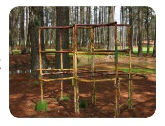
Equipment is mostly damaged to the point that use is limited or not possible, some pieces may pose safety hazards to users, footings are exposed, unstable, and/or severely damaged. Instructional Signage is no longer legible, is structurally unsound, or missing completely. Paths/Ground Surfaces are uneven, present trip hazards, allow water to pool, and limit access.
